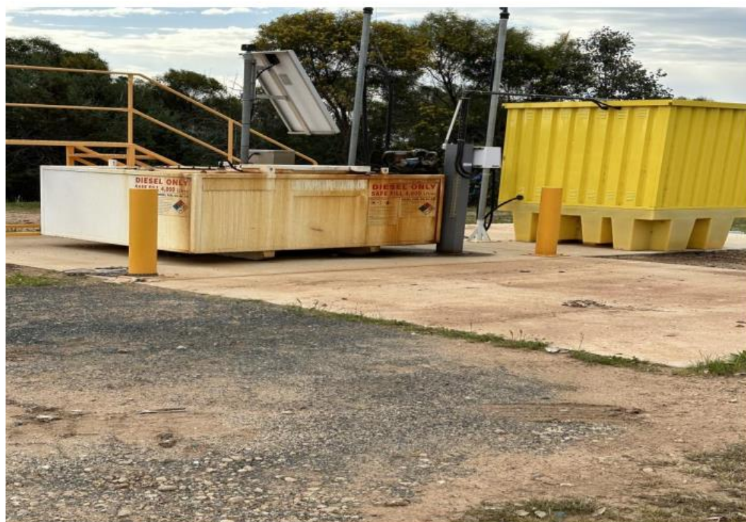
Figure 4-43: Self bunded diesel tank (Water Technology 2023)
