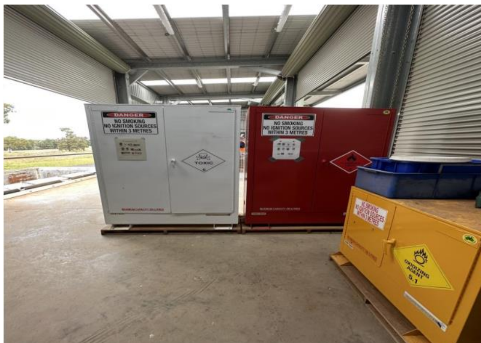
Figure 4-45: Hazardous Chemicals Storage Water Technology 2023)
