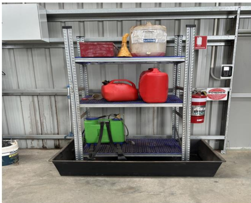
Figure 4-44: Stored chemicals with bunding (Water Technology 2023)
